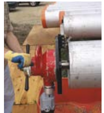
SDB pipe end preparation
